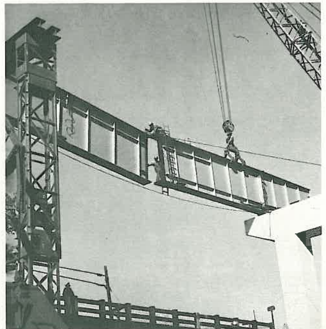
Setting the first overhead girders in place.
