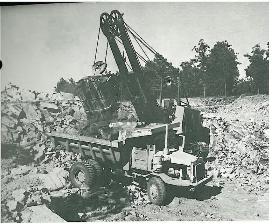
Rock is blasted loose and hauled away.
